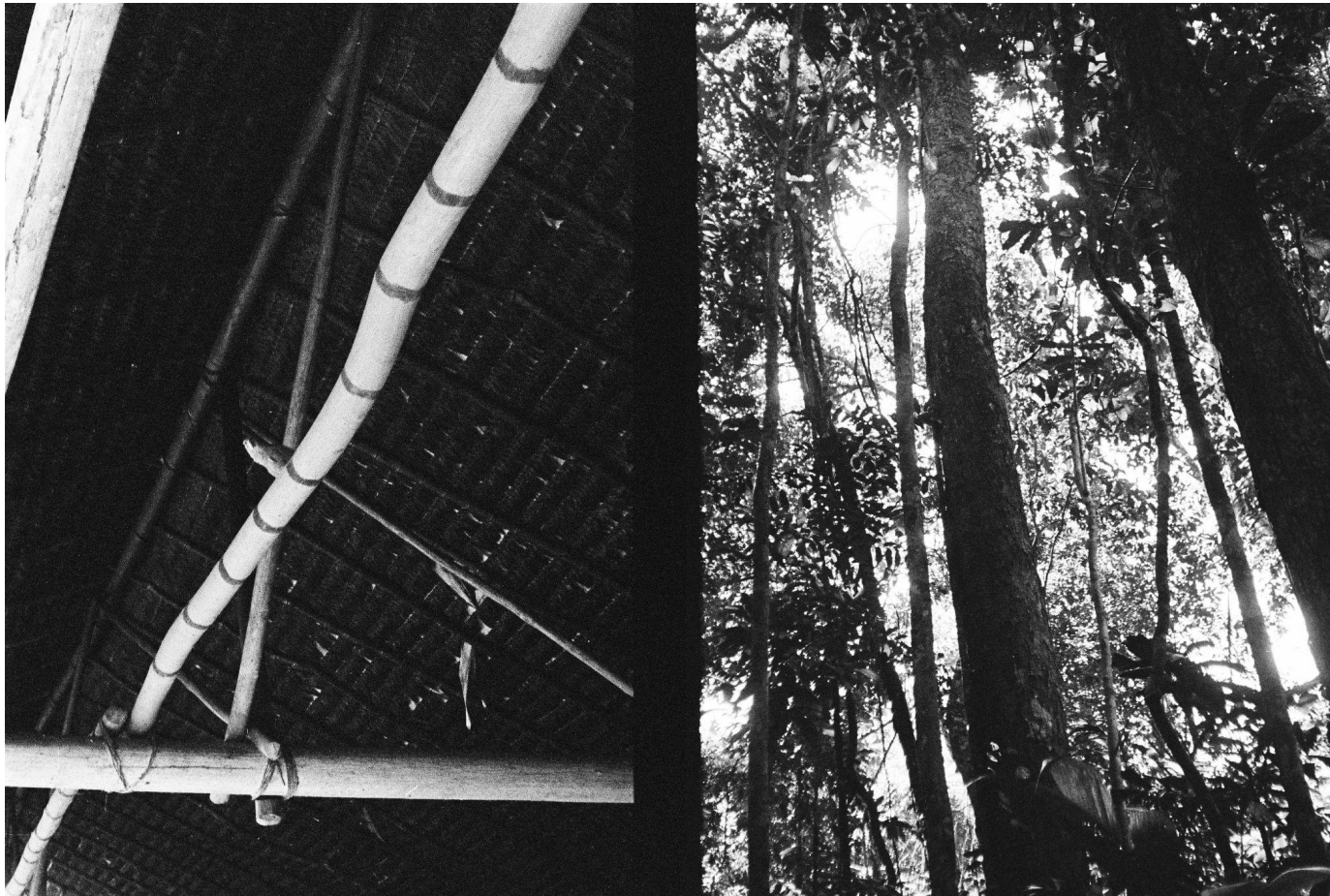
On the left, detail of a ceremonially painted wood beam, tied in the main wood structure with vine, and the soot darkened roof of a traditional house, owned by the leader of the Pukima Beira village at the upper river.
