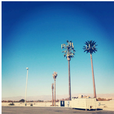
1 Invisible infrastructures. Camouflaged antenna in the form of a palm tree.
