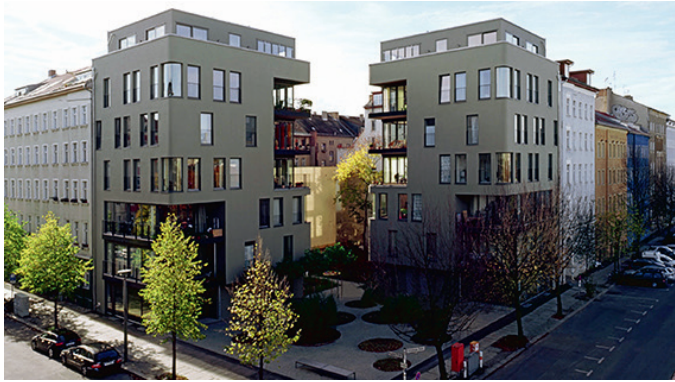
Fig. 2 North-oriented corner site between Schönholzerstrasse and Ruppiner Strasse
