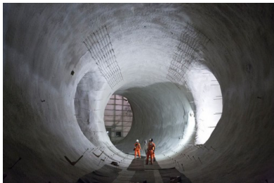
4 Cross rail underground infrastructure in London.
